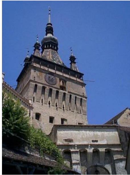
Citadel Clock Tower in Sighisoara
